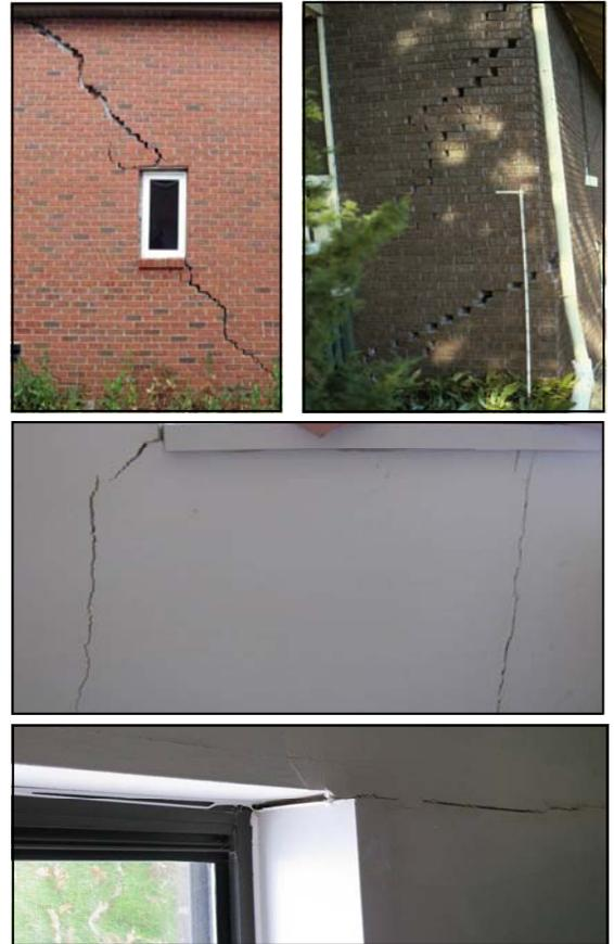
FIGURE 1 EXAMPLES OF AESTHETIC DAMAGE
