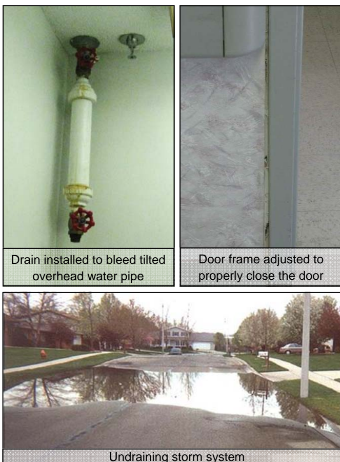
FIGURE 2 EXAMPLES OF FUNCTIONAL DAMAGE
