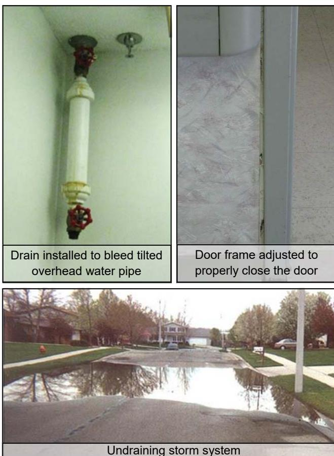
FIGURE 2 EXAMPLES OF FUNCTIONAL DAMAGE
