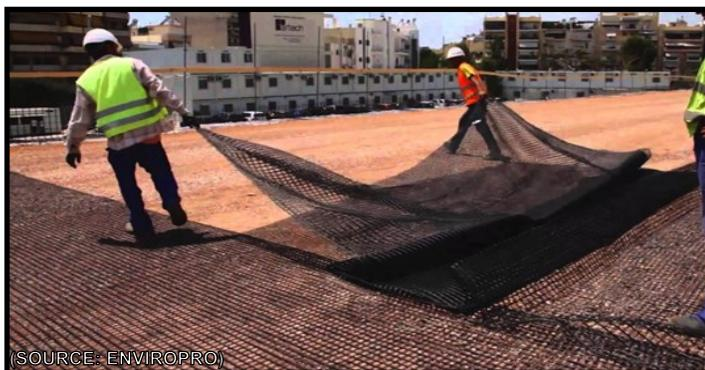
FIGURE 2 PLACEMENT OF GEOGRID OVER COMPACTED CONTROLLED FILL
