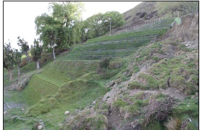
FIGURE 4: REINFORCED SOIL SLOPES
