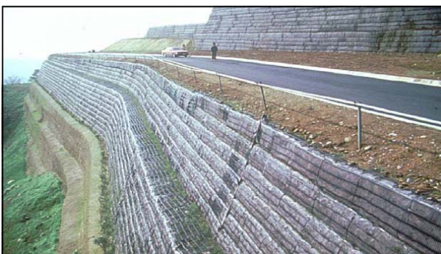
FIGURE 2: APPLICATION OF REINFORCED SOIL WALL IN A ROAD CONSTRUCTION PROJECT
